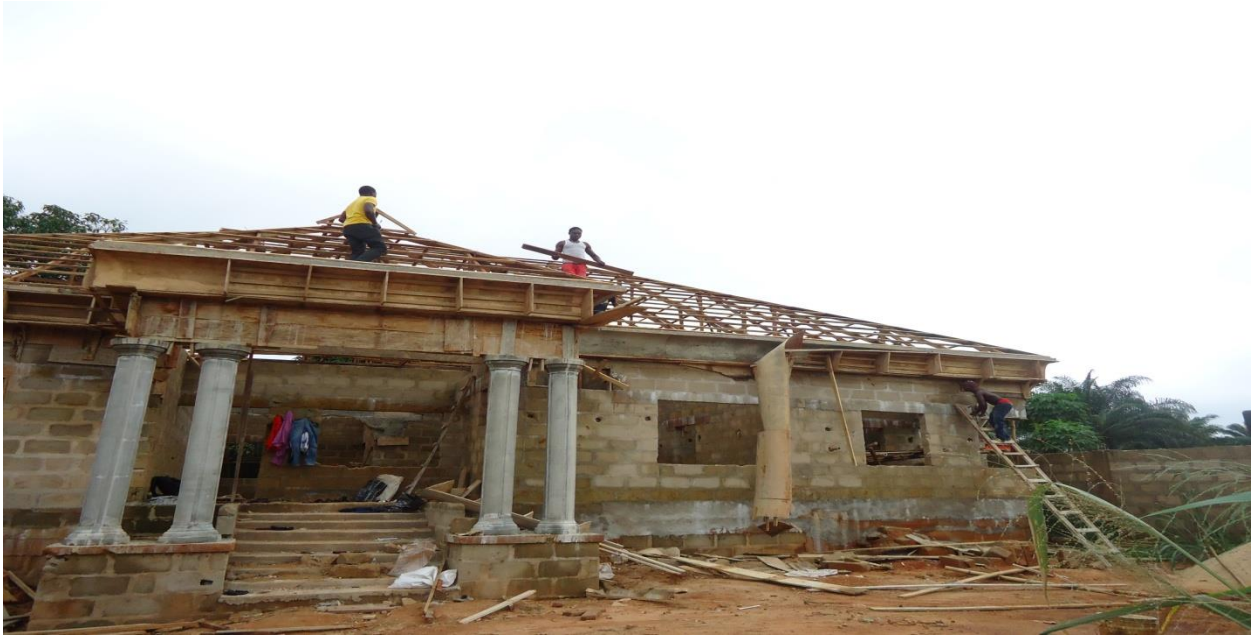
Roof Construction of Arben Medical Laboratory
