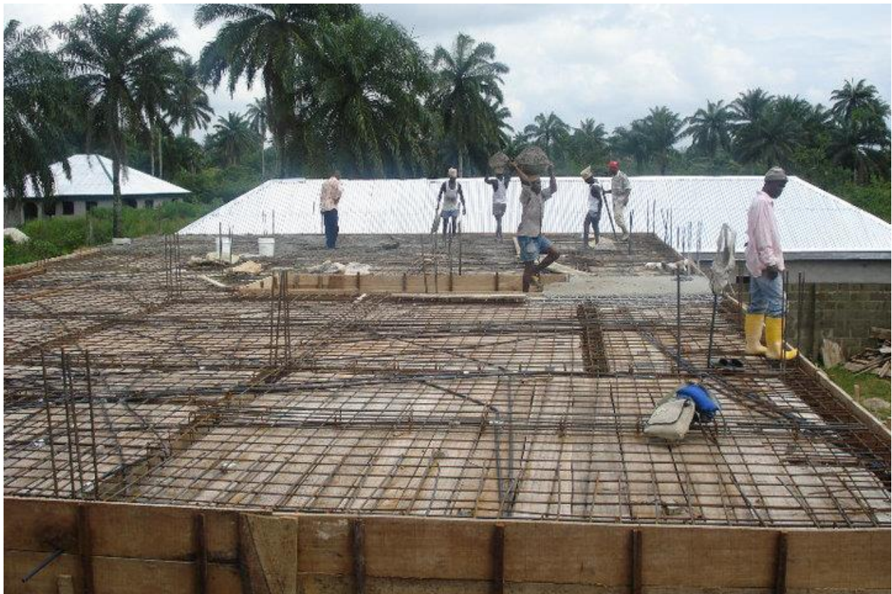
RCCG Office complex construction @ decking level
