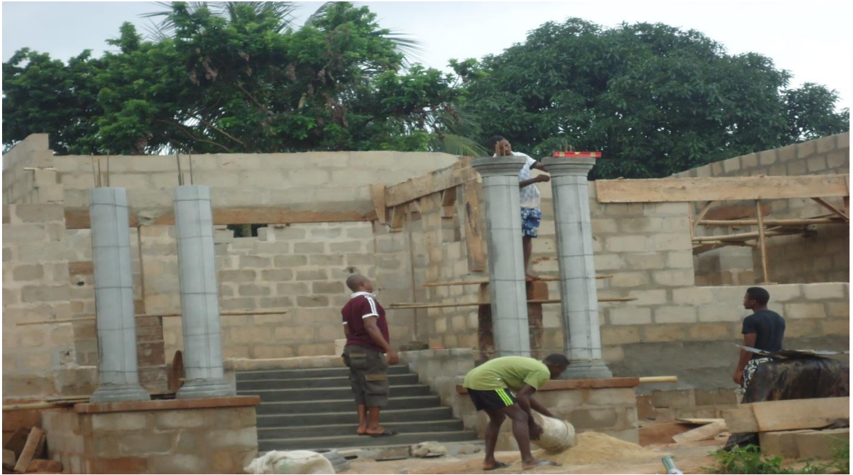
Construction of Arben Medical Laboratory
