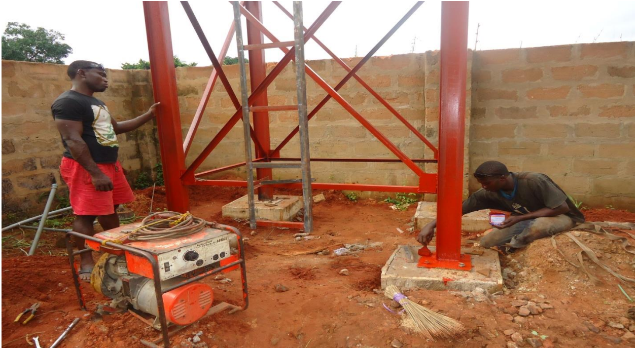
Over head tank stand base
