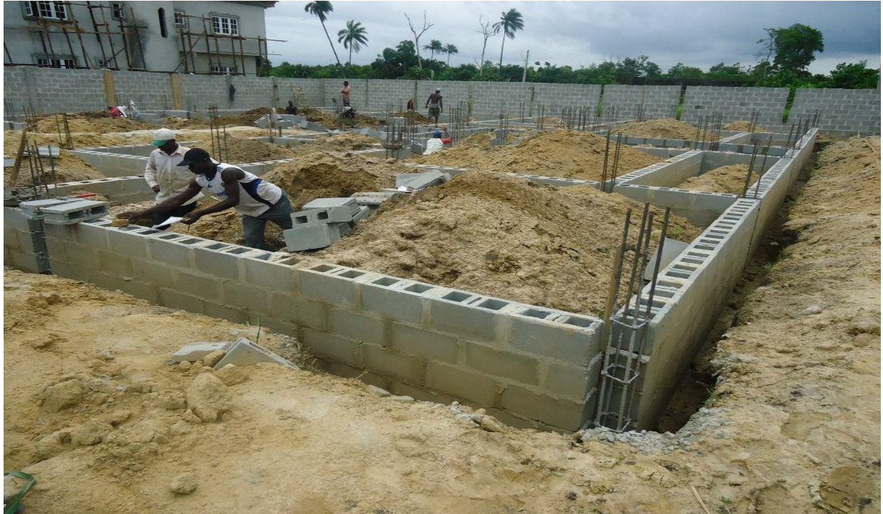
RCCG Office complex construction @ Foundation
