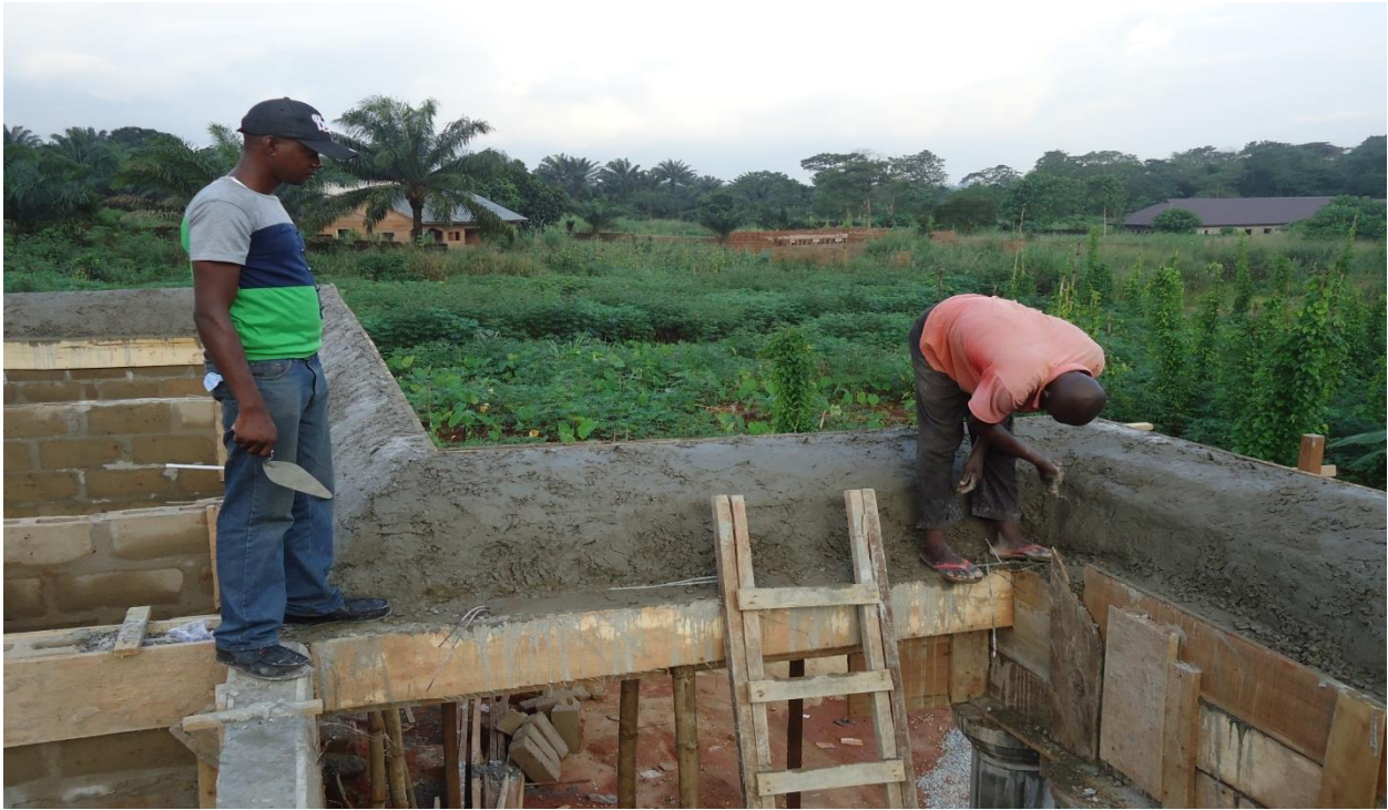
Parapet Construction of Arben Medical Laboratory
