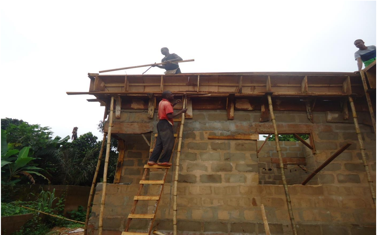
Parapet Construction of Arben Medical Laboratory
