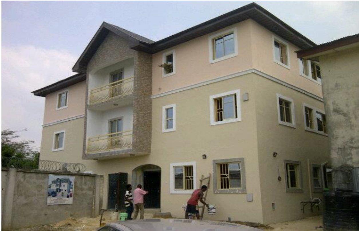
RCCG Office complex construction @ finished level
