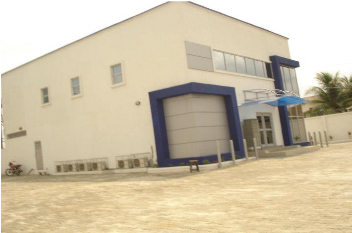
1st bank finished
