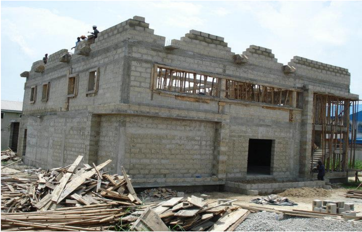
1st bank building construction work in progress
