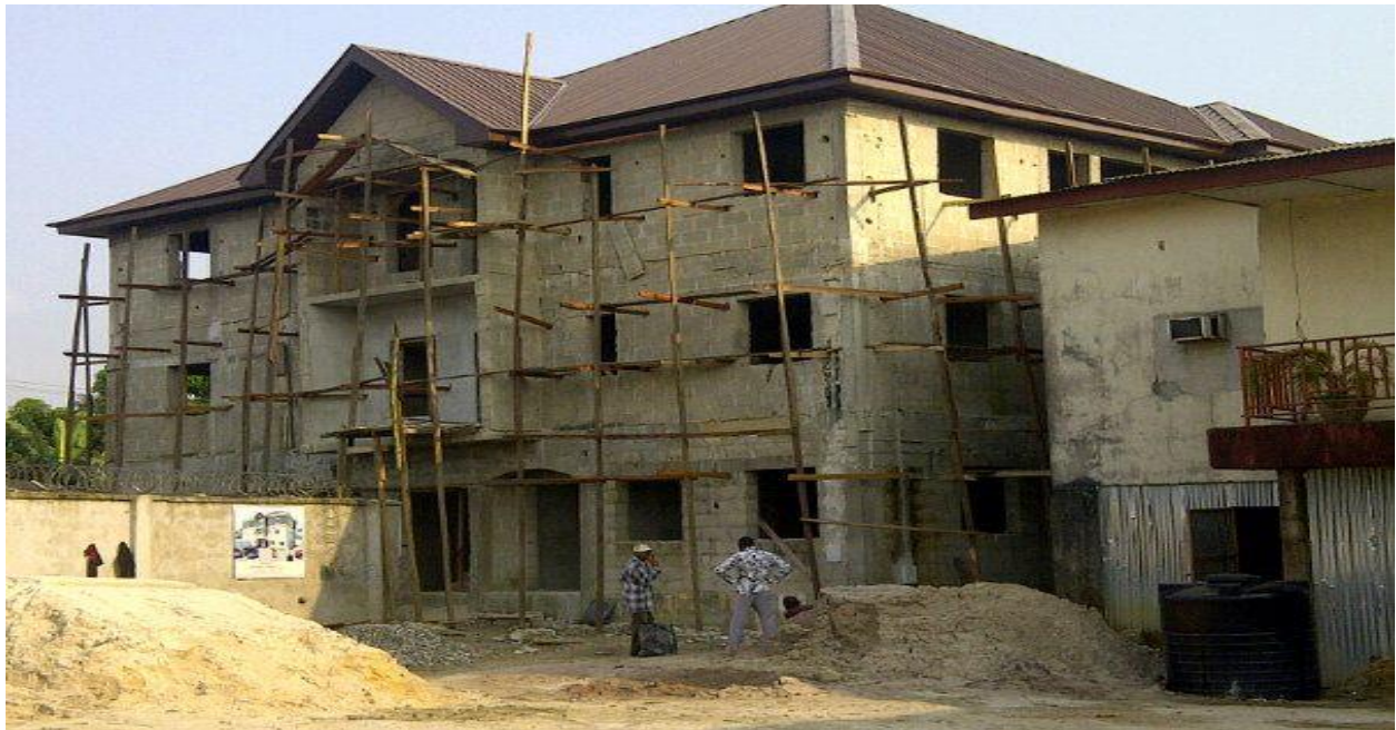
RCCG Office complex construction @ roof level
